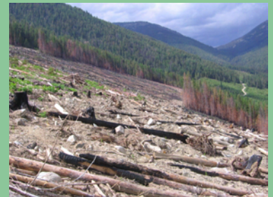
Atco rehabilitates unneeded roads by complete recontouring. This is done to minimize the losses of productive forest land to roads and to reduce the risk of future landslides and soil erosion resulting from bare road surfaces. In this harvested area, which had been burned in August 2006 by a wildfire, the recontoured road shows up well as the area in the centre of the photo which is much lighter in colour than the surrounding burnt ground.
